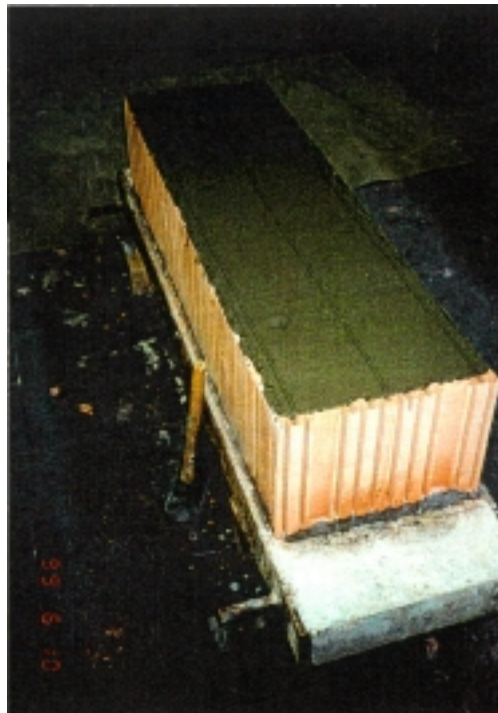
Picture 4: Cover up thin layer mortar 15 minutes after application
