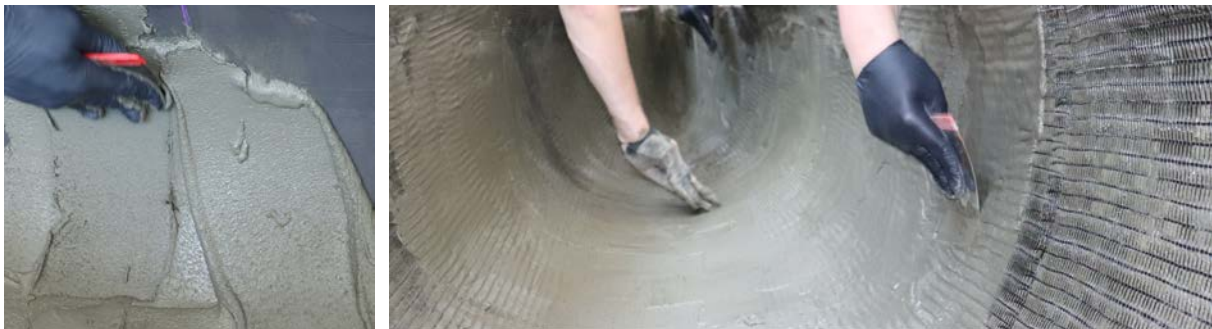
(a) as a first layer (b) as a second layer on first layer and textile reinforcement
