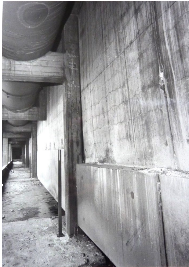
Fig. 6: Outer side wall of the furnace (from [3])
