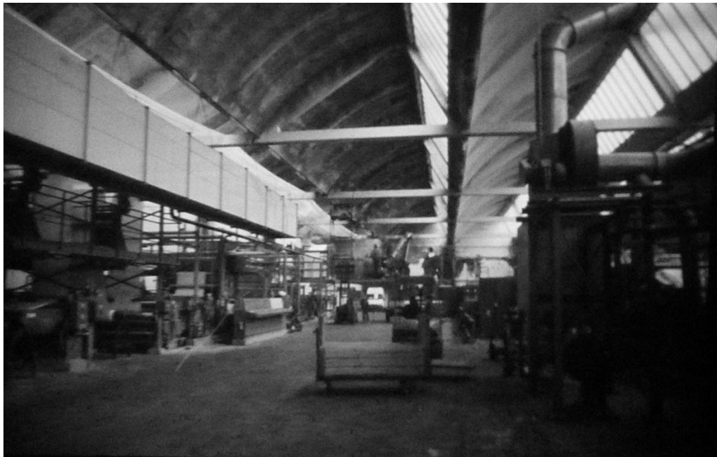
Fig. 8: The sheds resting on the trussed girder
