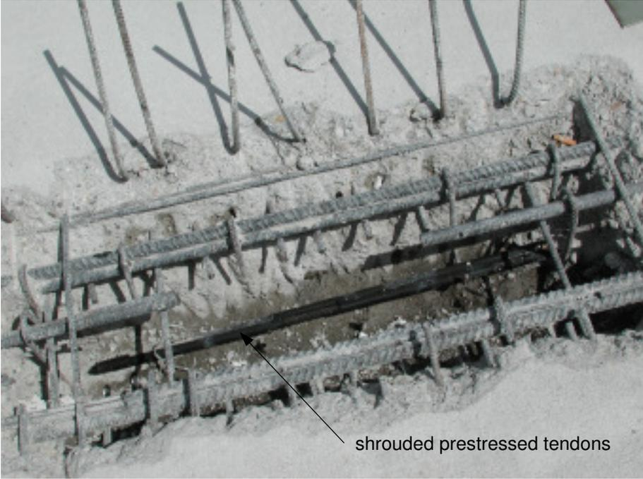
*Fig. 4: stemmed surface of the slab in the area of tendons (axis 204)*
