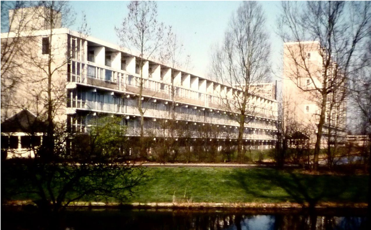
Fig. 2: Building after removal of several stories
