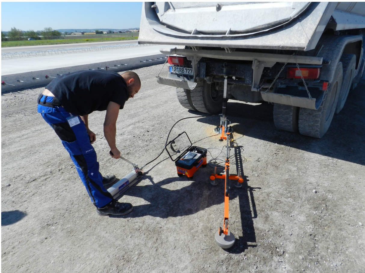
Fig. 4: Measurement of the load-bearing capacity of the hydraulically bound base layer
