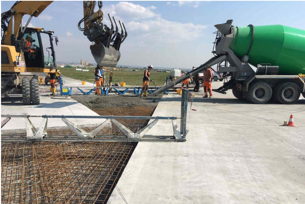
Fig. 9: Manual concrete placement
