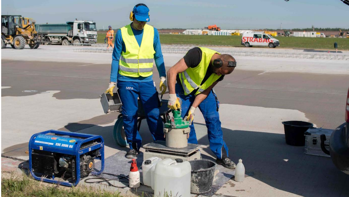
Fig. 10: Acceptance testing at the paving site
