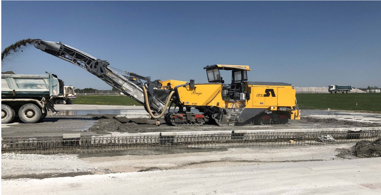
Fig. 3: Milling machine for removing the 40 cm thick concrete slabs
