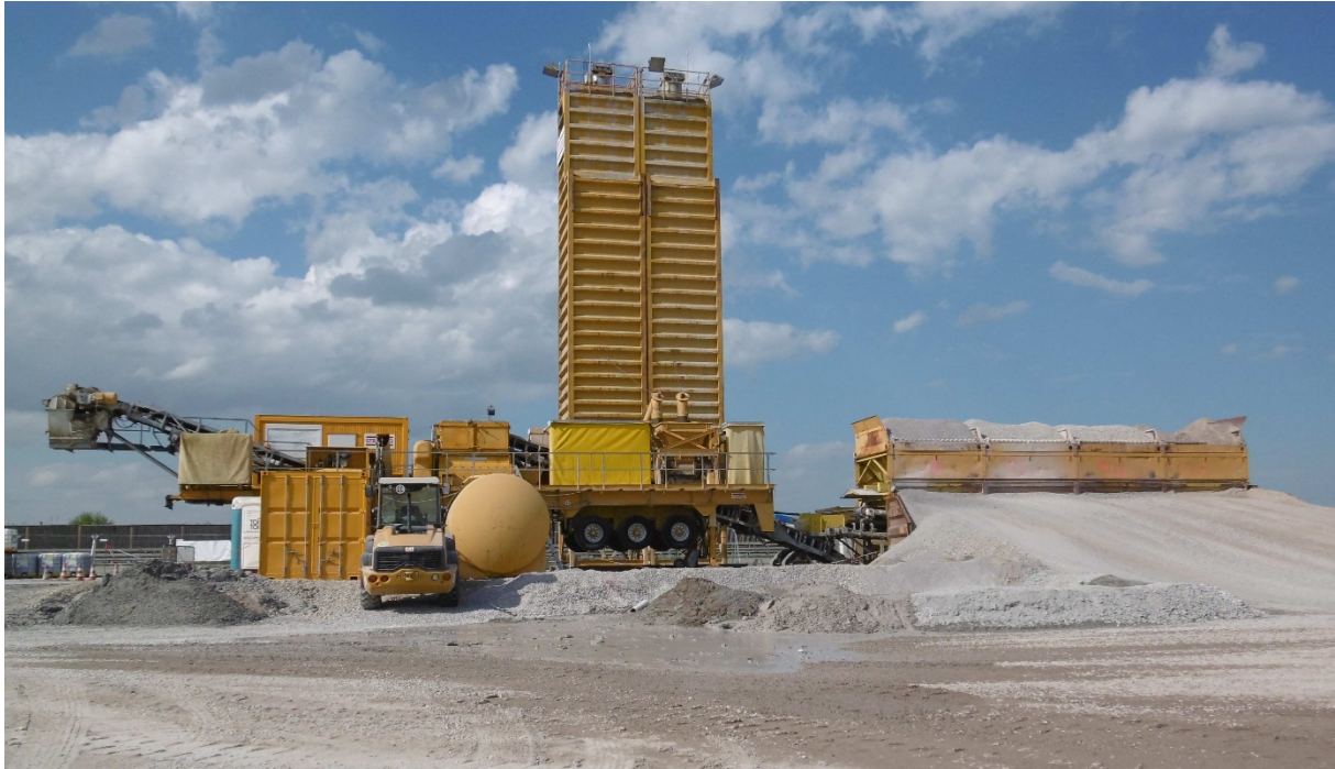
Fig. 6: Mobile continuous mixer type for the paver concrete
