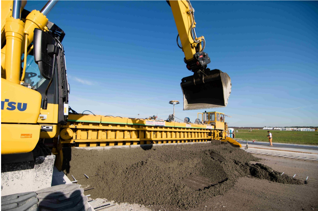
Fig. 7: Slipform paver. Distribution of concrete with an excavator
