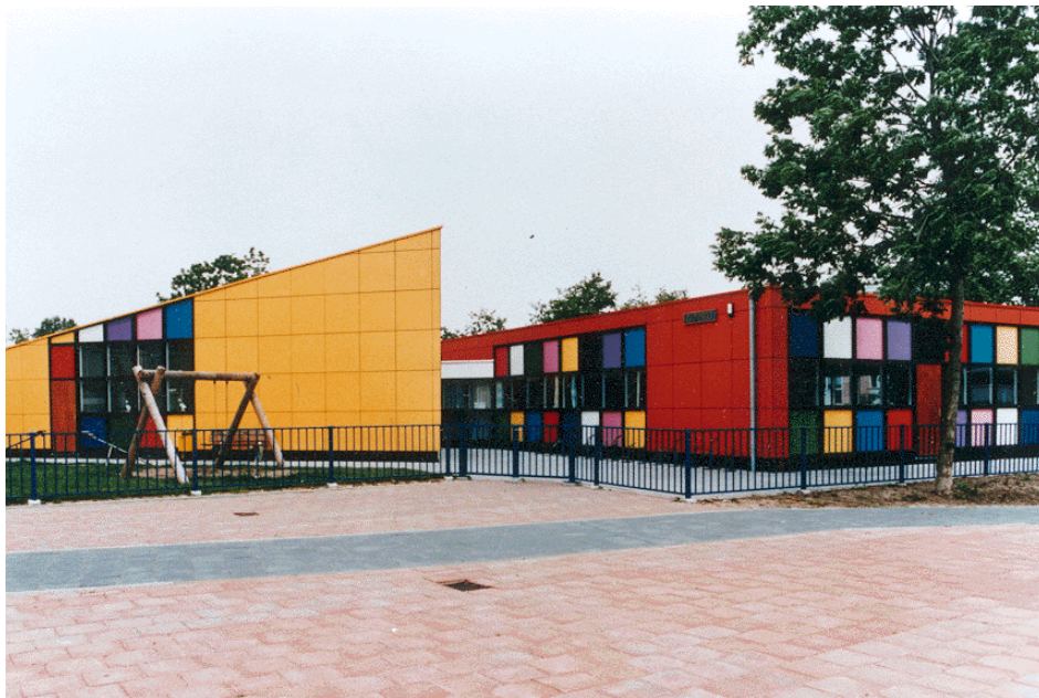
Fig. 1. Single-storey building as an example for the use of decorative facade panels
