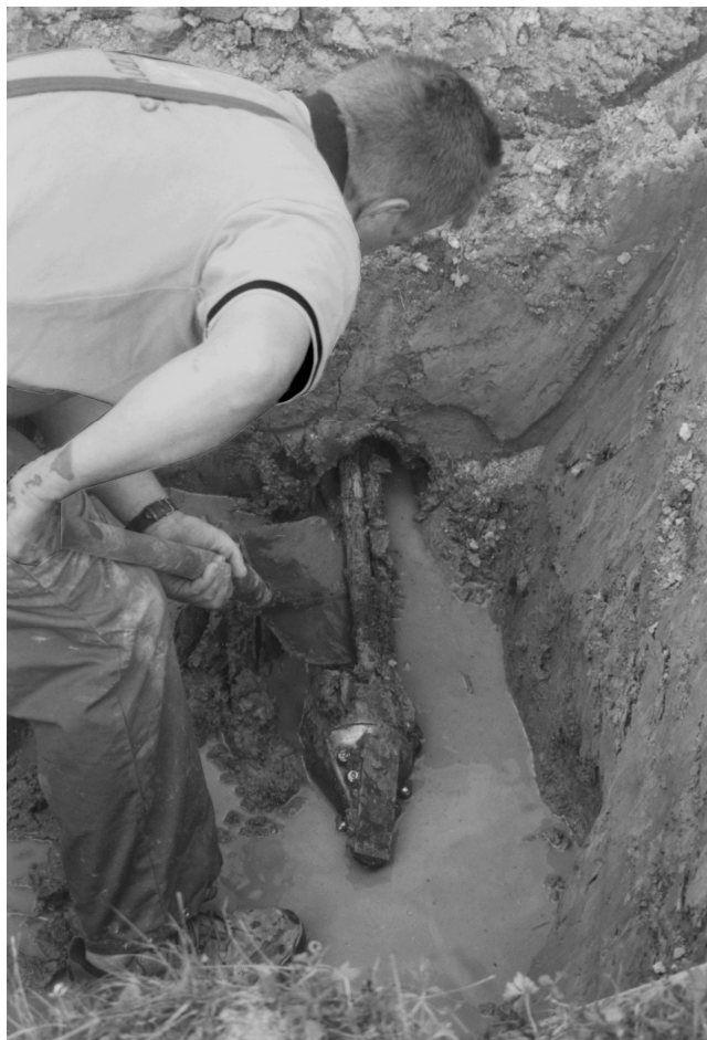
Figure 5: Digging for a spool-drilling head in a manhole at the ending-point of a steered horizontal boring. (Tracto-Technik Company, System Grundopit).
