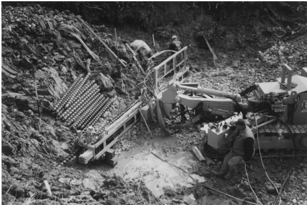
Figure 1: Nonsteerable horizontal screw-boring for the installation of 3''-steel-pipes. The slope-draining project at the Thanheimer Steige, L 360, Baden-Württemberg, May 2006.
