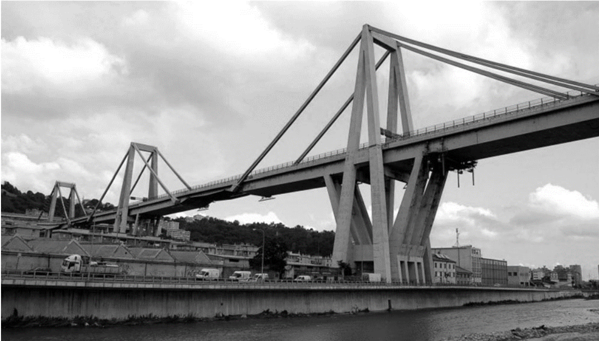
Fig. 3: Polcevera viaduct in Genoa [4]
