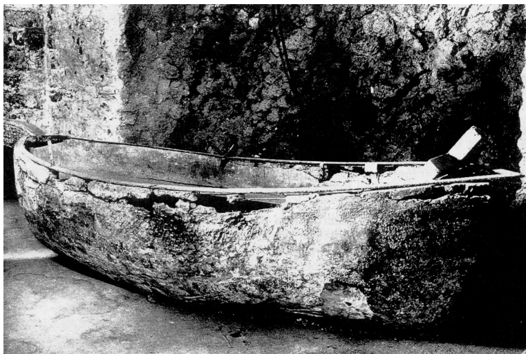
Fig. 1. Lambot's ship of 1848 made of concrete [1]
