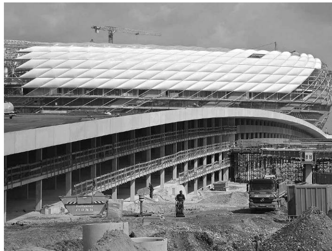
Figure 7: Side view of the multi-storey car park (source: www.allianz-arena.org )
