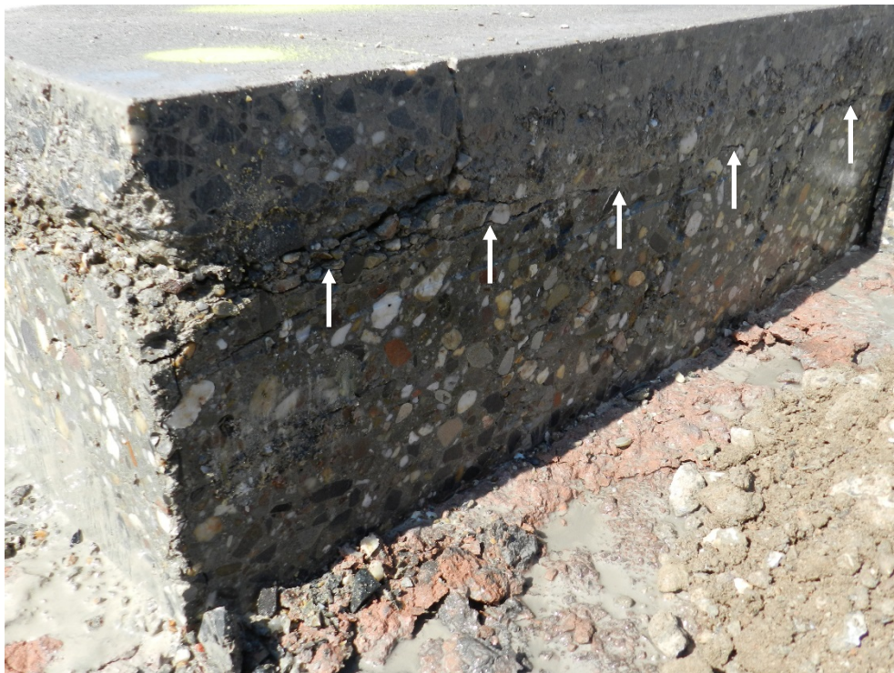
Fig. 2: Horizontal cracks related to corner fracture in Fig. 1
