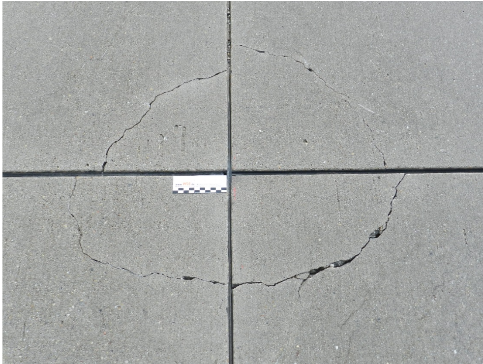
Fig. 1: Corner fracture
