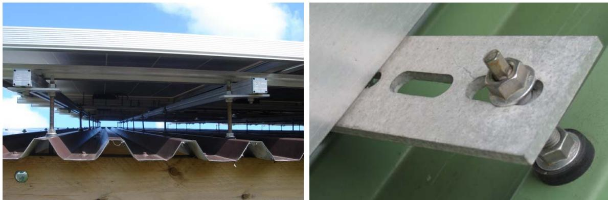
*Fig. 2: Photovoltaic modules mounted on a trapezoidal sheet metal roof (left) and mounting detail (right): flat profile made of AlMgSi 0.7 and fastening system made of 1.4301*
