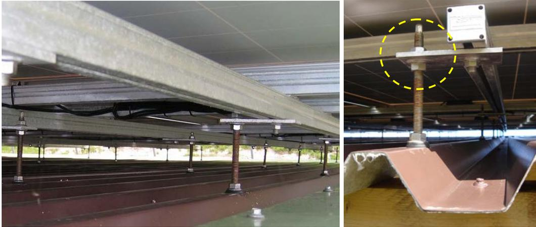
*Fig. 7: Substructure of the photovoltaic system and detail marked with a yellow circle*
