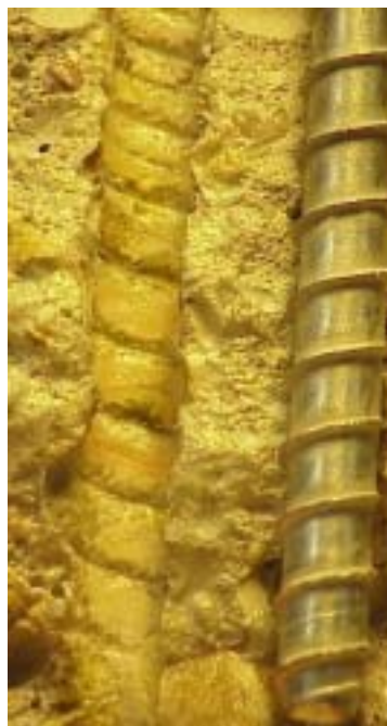
Figure 2: Concrete screw and a thread cut into the wall of the drilled hole [9]
