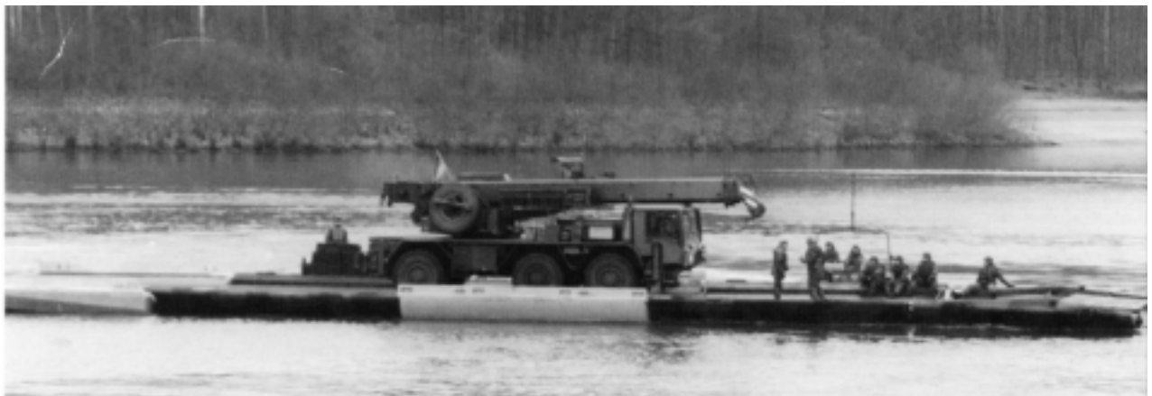
Fig. 1: Floating bridge in service
