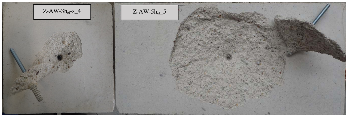
Fig. 3: Mixed failure mode and brick cone breakout
