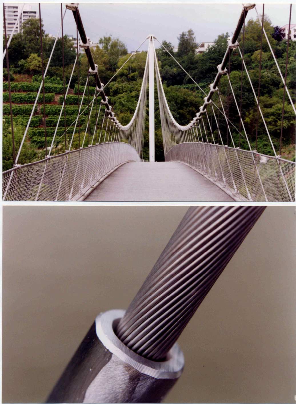
Fig. 5: Open spiral strands of a suspension bridge with suspended reinforced concrete foot-bridge
