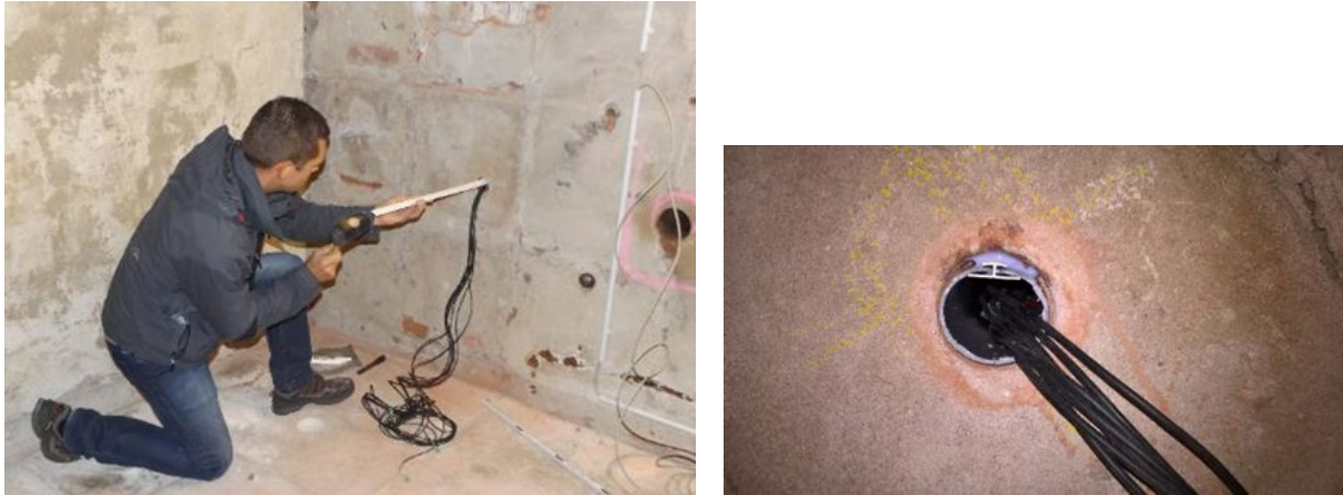
Fig. 5: left: Driving in the clamping profile, right: Installation condition after clamping
