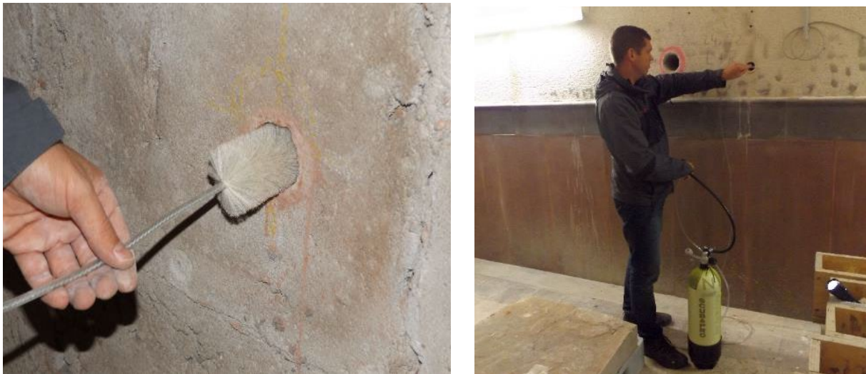
Fig. 4: left: Cleaning out the boreholes, right: Blow out with compressed air
