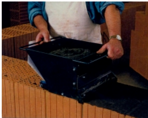
Picture 3: Apply of cover up thin layer mortar with a mortar roll
