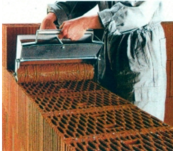
Picture 1: Apply of thin layer mortar with a mortar roll
