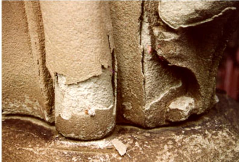
*Fig. 1 Typical deterioration of sandstones scaling on the surface and beneath it sandy decay*
