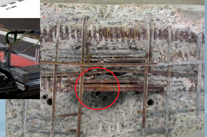
Fracture of prestressed tendon in a bridge
